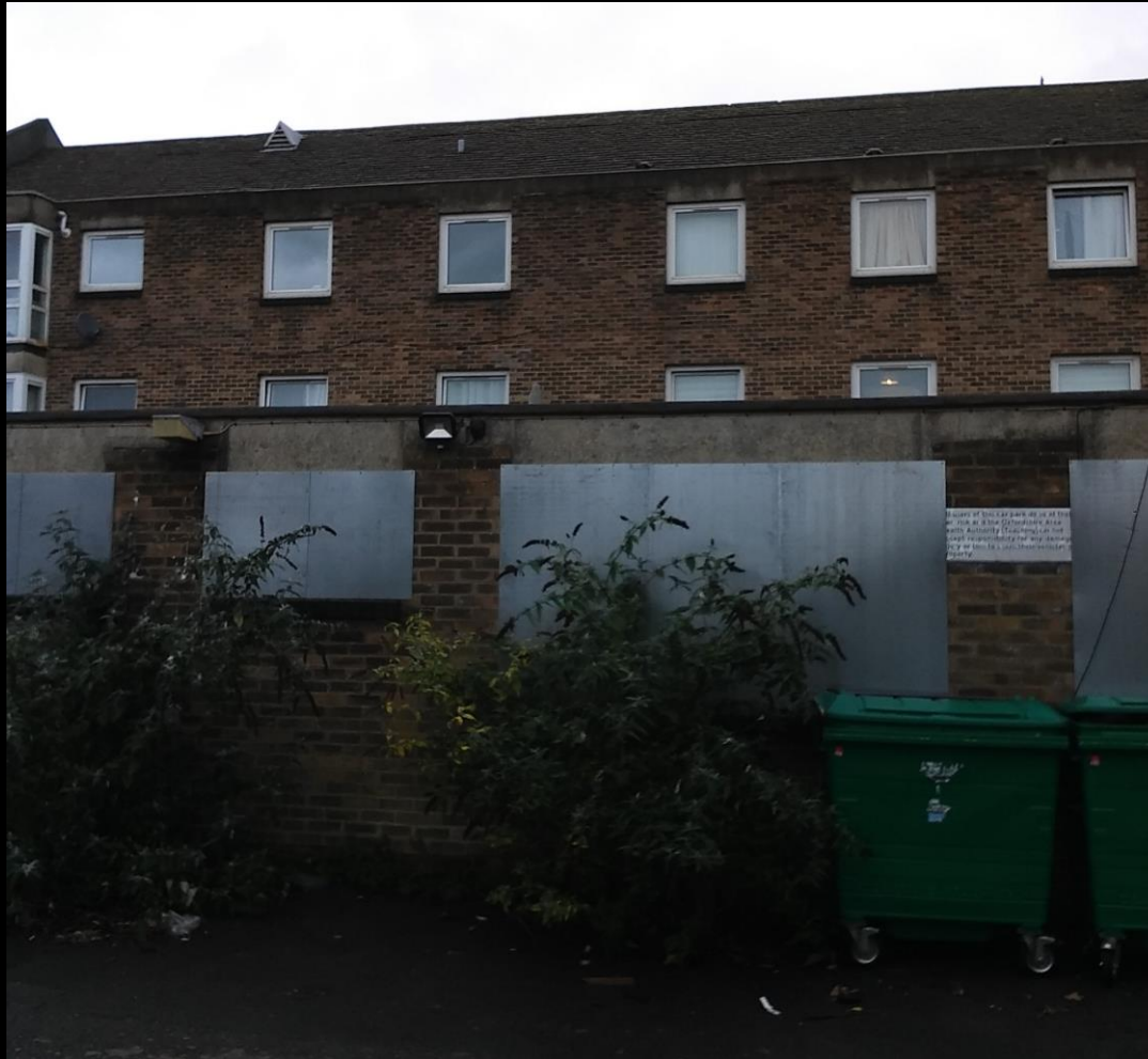
View of north east elevation from Venables Close
