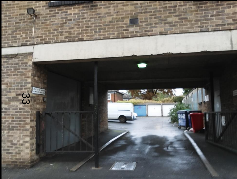
View north east into existing car park
